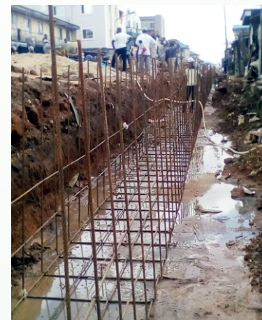
ALIGNMENT OF RE-ENFORCEMENT BARS, ADEBULE STREET, MUSHIN.
