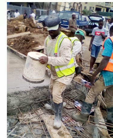
CASTING OF SLAB OF CROSS CULVERT, PALM AVENUE/BUARI, MUSHIN.
