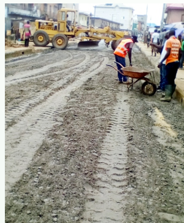
GRADING OF STONE BASE AT ANIPELE STREET, MUSHIN.
