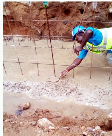
CASTING OF 150MM THICK BASE OF DRAINAGE BUARI, MSUHN
