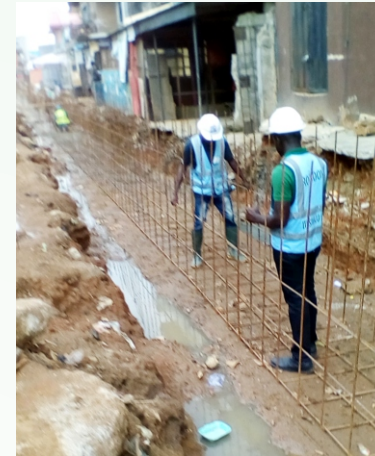
ALIGNMENT OF RE-ENFORCEMENT BARS AT BUARI STREET, MUSHIN.
