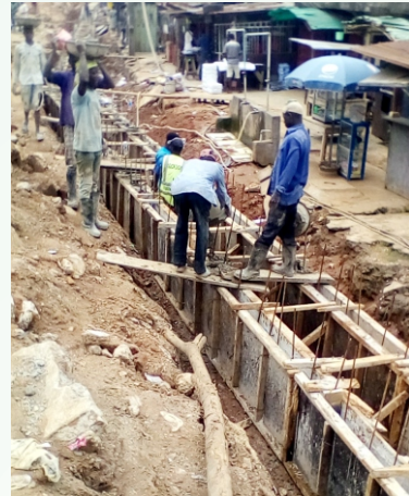
CASTING OF 150MM THICK WALL OF DRAINAGE AT BUARI STREET, MUSHIN.
