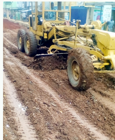
GRADING OF LATERITE AT ADEBULE STREET, MUSHIN.
