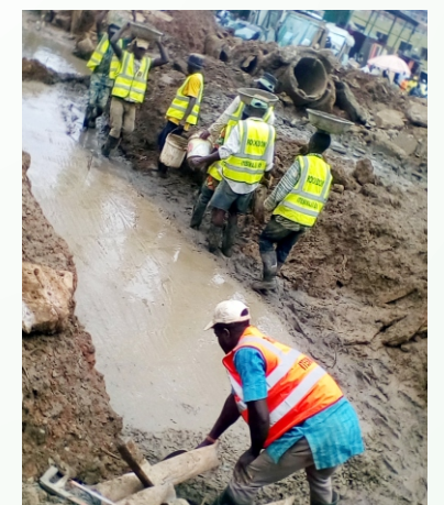
CASTING OF 50MM THICK BLINDING, PALM AVENUE/BUARI, MUSHIN.
