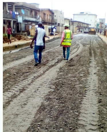
GRADING OF STONE BASE AT BUARI STREET, MUSHIN.
