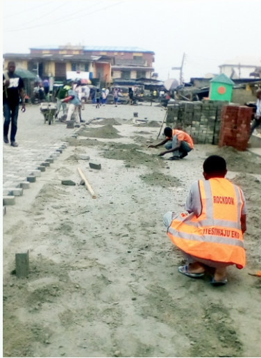
TAKING OF LEVEL FOR LAYING OF INTER-LOCKING STONES IKALE STREET, ITIRE-IKATE,
