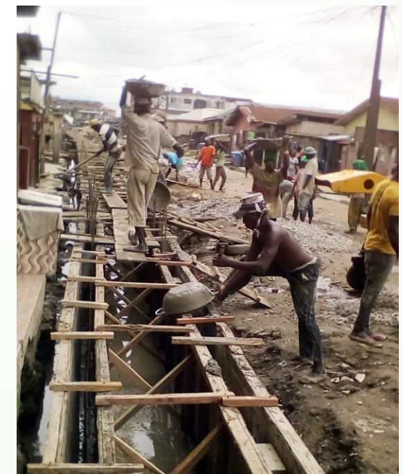
CASTING OF 150MM THICK WALL OF DRAINAGE AT IKALE STREET, ITIRE-IKATE
