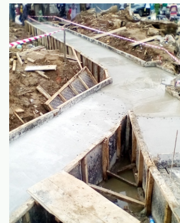
CASTING OF 150MM THICK WALL FOR CROSS CULVERT AT PALM AVENUE/BUARI, MUSHIN.
