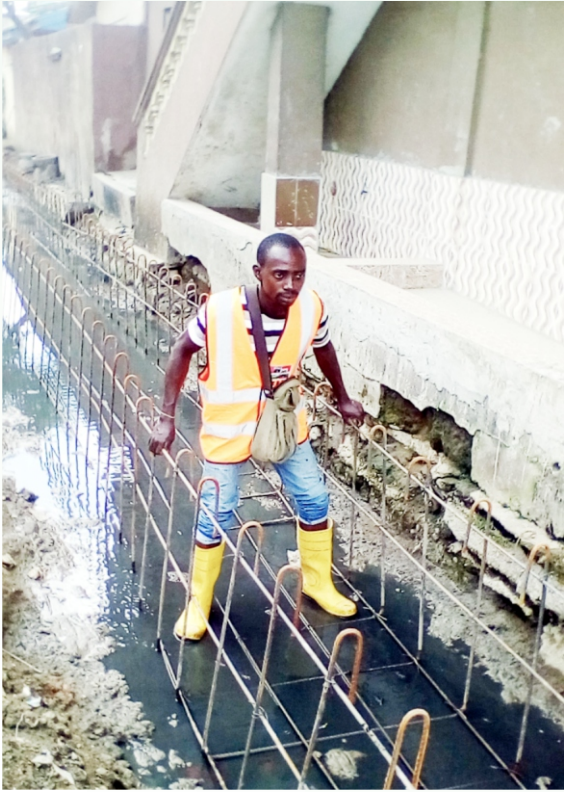
ALIGNMENT OF RE-ENFORCEMENT, IKALE STREET, ITIRE-IKATE.
