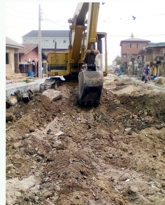
SCLARIFICATION PROCESS AT IKALE STREET, ITIRE-IKATE
