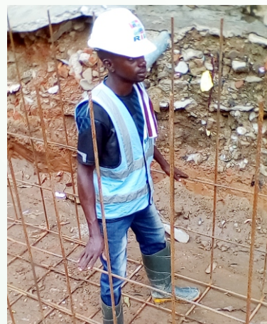
ALIGNMENT OF RE-ENFORCEMENT BARS, ANIPELE STREET, MUSHIN.
