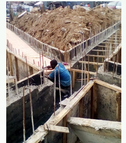
PREPARING OF FORM WORK BY CARPENTER FOR CROSS COVER SLAB AT PALM AVENUE/BUARI, MUSHIN.
