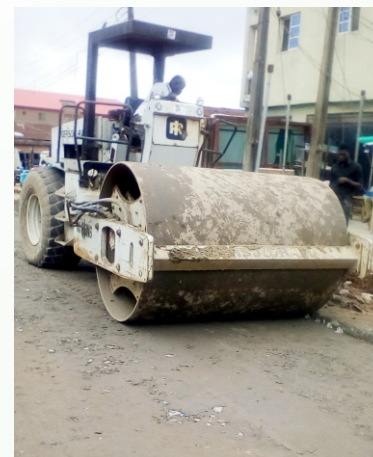
ROLLING OF STONE BASE AT ADEBULE STREET, MUSHIN.
