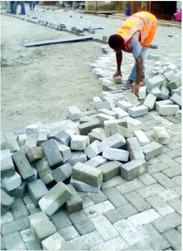
LAYING OF INTER-LOCKING STONES IKALE STREET, ITIRE-IKATE,
