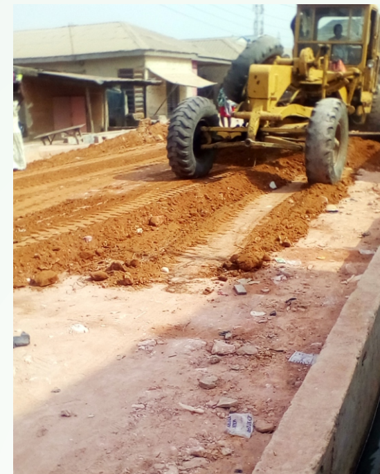
GRADING OF LATERITE ON SITE AT IKALE STREET, ITIRE-IKATE.
