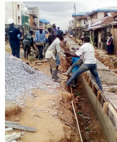
CASTING OF 150MM THICK WALK WAY, BUARI STREET, MUSHIN.
