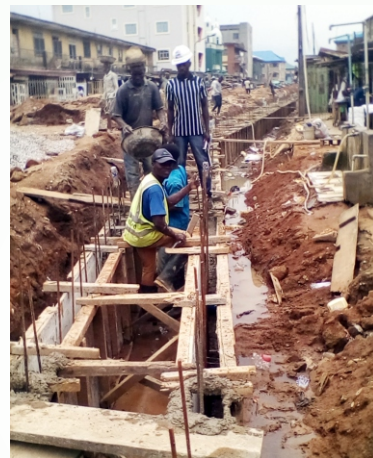
CASTING OF 150MM DRAINAGE WALL, ANIPELE, MUSHIN.
