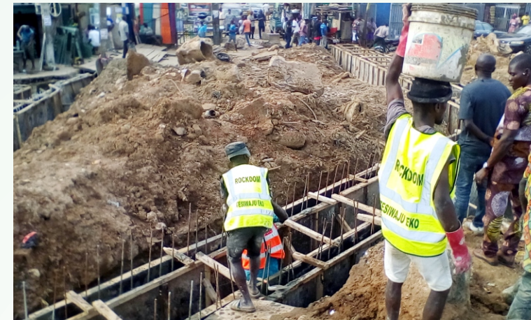
CASTING OF 150MM THICK WALL FOR CROSS CULVERT AT PALM AVENUE/BUARI, MUSHIN.
